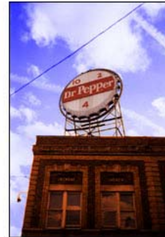
Increased blue in sky, applied complement orange 15% to sign, 40% to building
